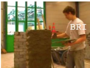
#1: BRI tries to throw cement on the wall with his trowel
