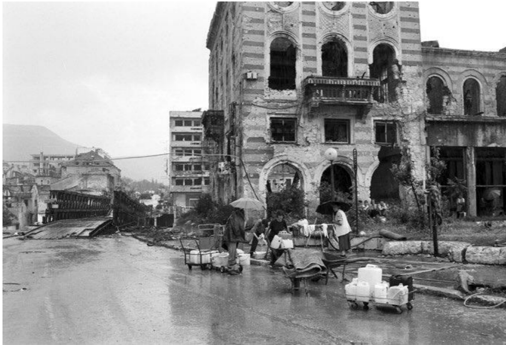
Collecting water in Mostar, Bosnia-Herzegovina, 1993. ICRC, Urban services during protracted armed conflict: a call for a better approach to assisting affected people , 2015, p.15
