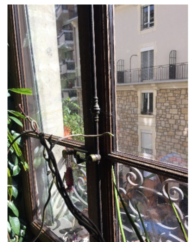
Picture 5. An old building's simple glazing window
