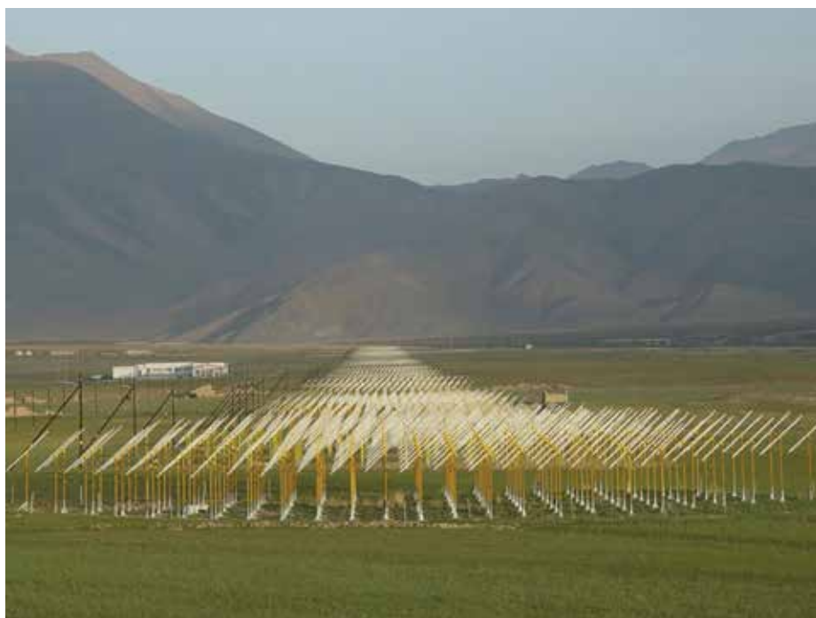
Figure 49 The Wulasitai Observing Station. Copyright © National Astronomical Observatories, Chinese Academy of Sciences
