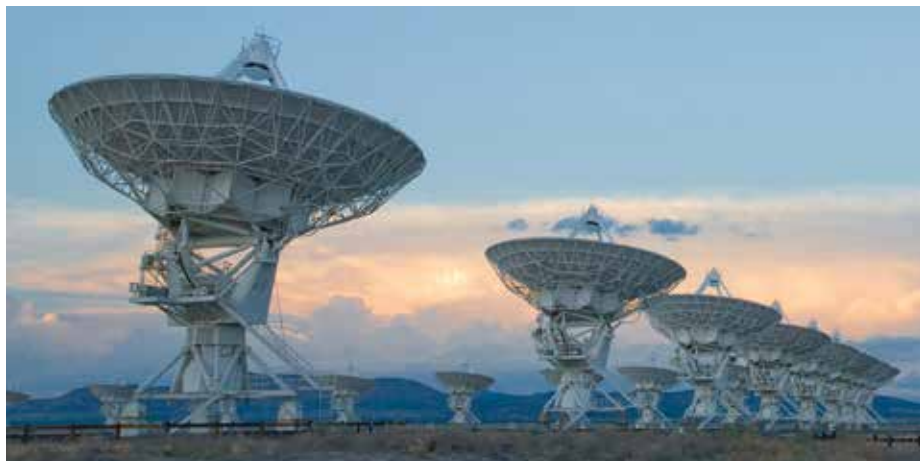
Figure 50 The Very Large Array (VLA) is a collection of 27 radio antennas located at the NRAO site in Socorro, New Mexico. Each antenna in the array measures 25 meters (82 feet) in diameter and weighs about 230 tons. Credit Alex Savello / National Radio Astronomy Observatory
