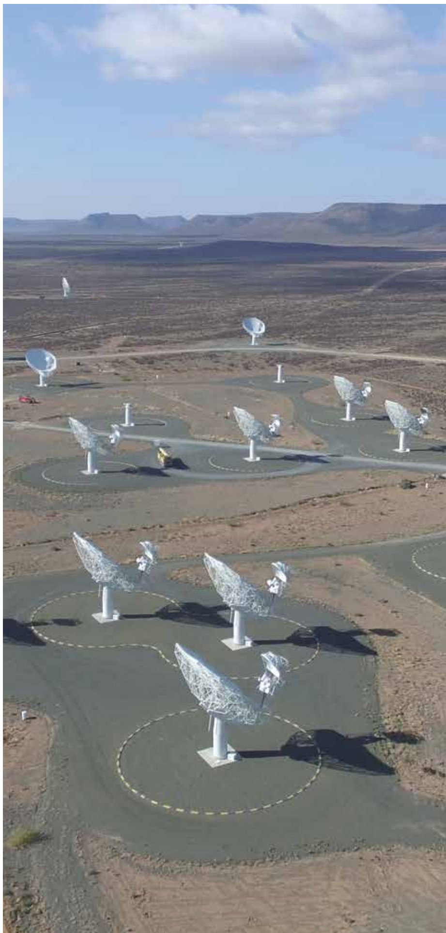
Figure 28 Aerial shot of the MeerKAT radio telescope before its launch in July 2018. These sunrise shots show the expanse of the telescope, which covers a baseline distance of 8 km. Credit : South African Radio Astronomy Observatory (SARAO)
