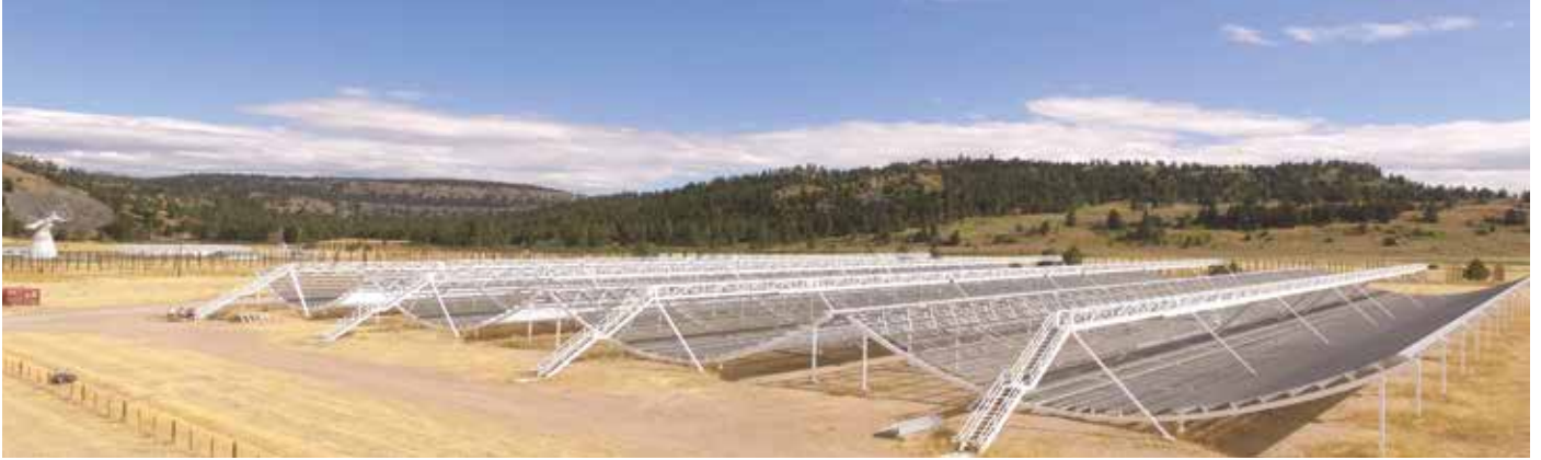
Figure 54 Image of the 4 cylinders and 1024 dual-polarized antennas of the CHIME telescope located at the Dominion Radio Astrophysical Observatory (DFAO), a national facility for astronomy operated by the National Research Council of Canada. Credit: chime-experiment.ca
