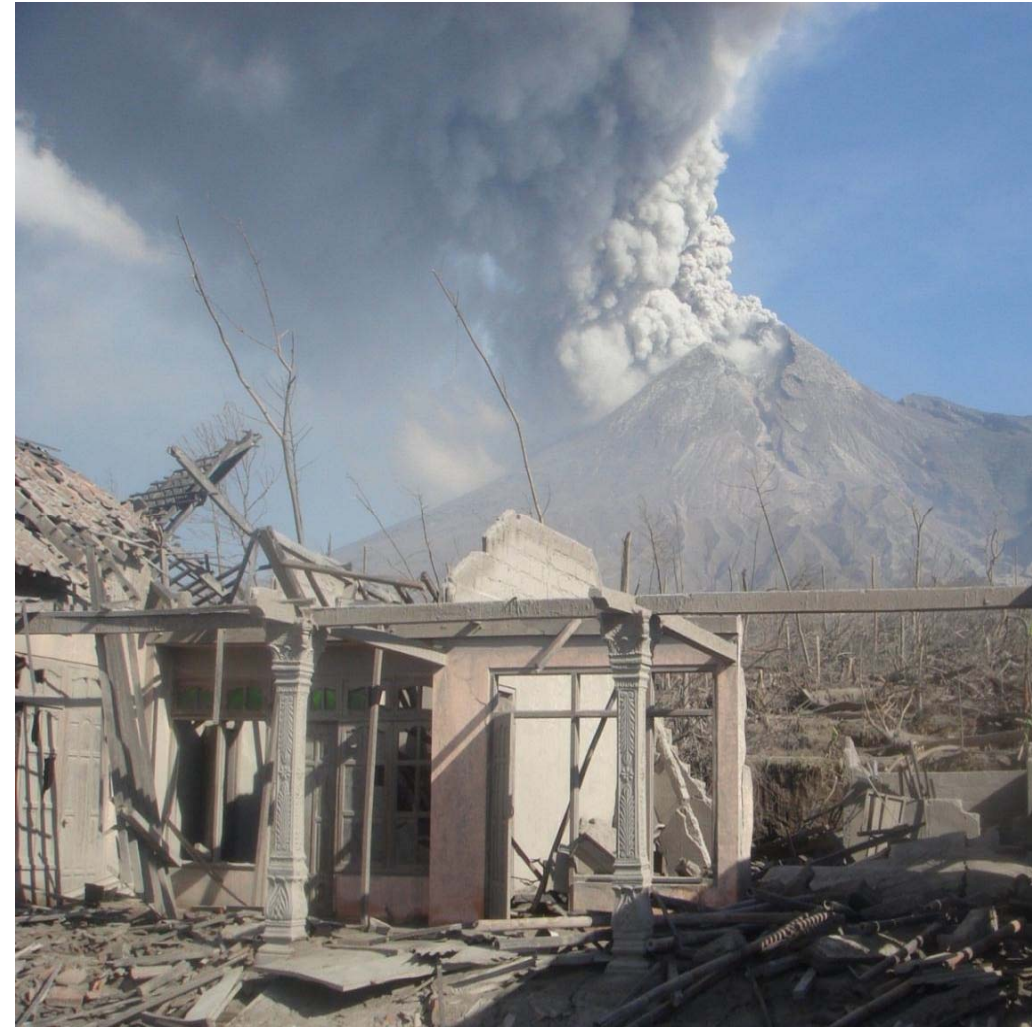
Damage to the village of Balerante, 5km from Merapi volcano during the October-November 2010 eruption [Photo: courtesy of Balerante village chief]
