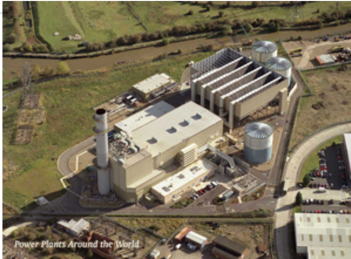
400-MW single-shaft combined-cycle block with GT26B gas turbine Enfield, Middlesex, 2000 (sold 2005 for 200 Mio. Fr)
