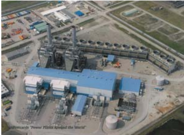
790 MW, 2+1 combined-cycle cogeneration plant with V94.3A gas turbines Rijnmond, Holland, 2004
