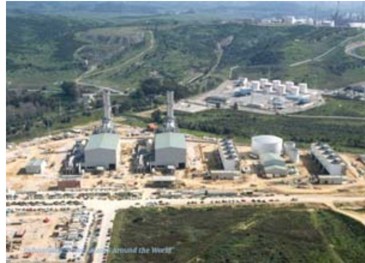
2 x 400 MW single-shaft combined-cycle blocks with GT26B gas turbines San Roque, Cadiz, 2002 (Spain)
