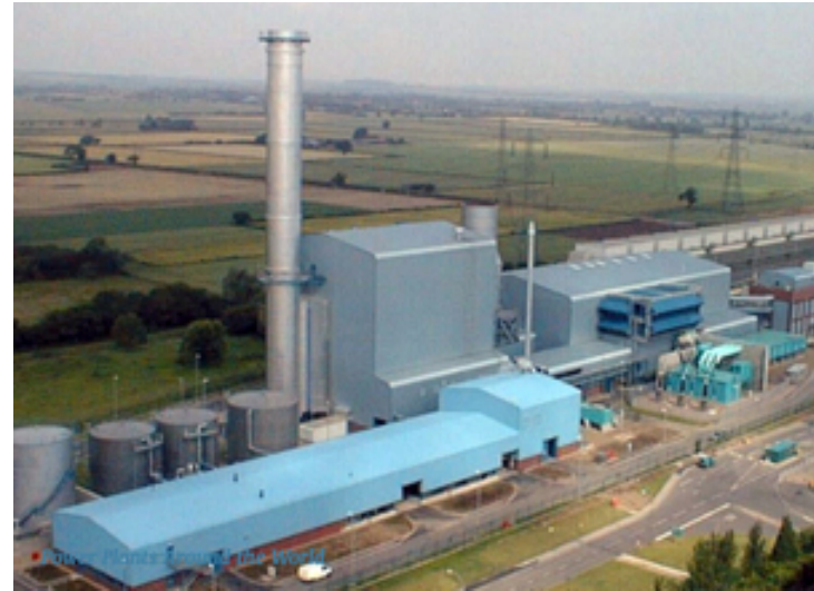
400-MW single-shaft combined-cycle block with V94.3A gas turbine Cottam CDC, Nottinghamshire, 1999
