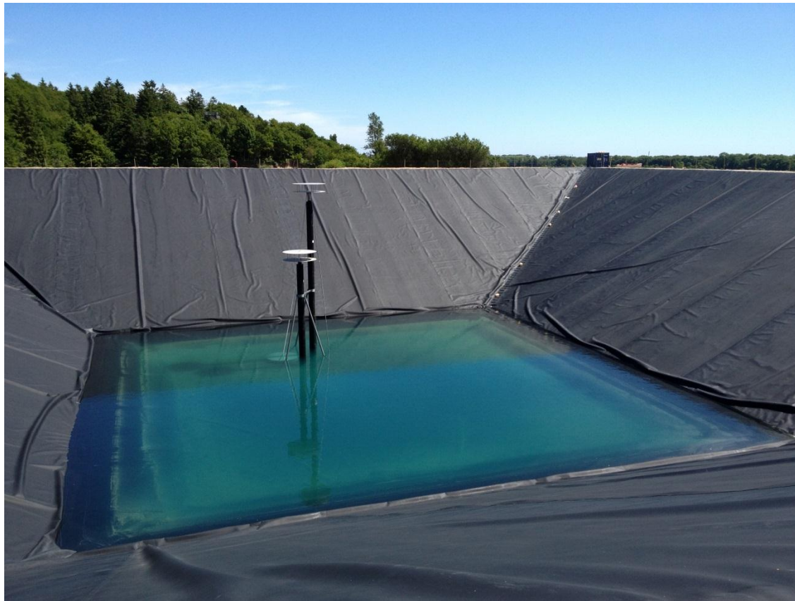
Dronninglund: 60,000 m 3 pit heat storage (under construction)
